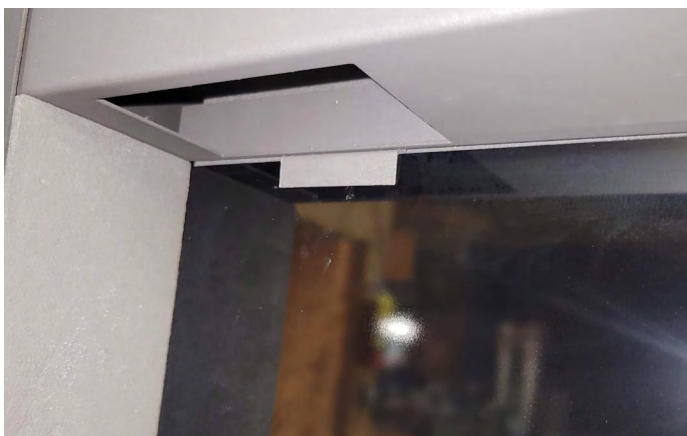
Figure 17.2.03: Glass retainer clip installed
