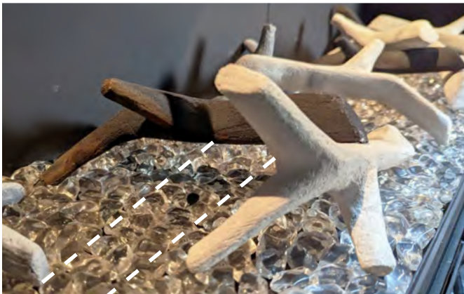
Figure 3.0.02: Use logs to bridge the burner.
